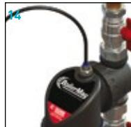
**CHEMICAL DOSING** Isolate boiler. Close isolation valves. Open drain valve to release air pressure (6). Close drain valve. Remove air vent screw (12) or fully remove air vent (13). Connect dosing device (14). Open outlet isolation valve. Apply dose (500ml max.). Close outlet isolation
